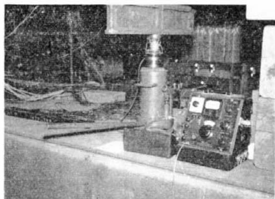
Fig. 3·6 Loading and Measuring Apparatus for Bending Moment
